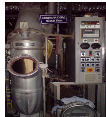
Fig. 1: Thies Winch Dyeing Machine (Germany)
