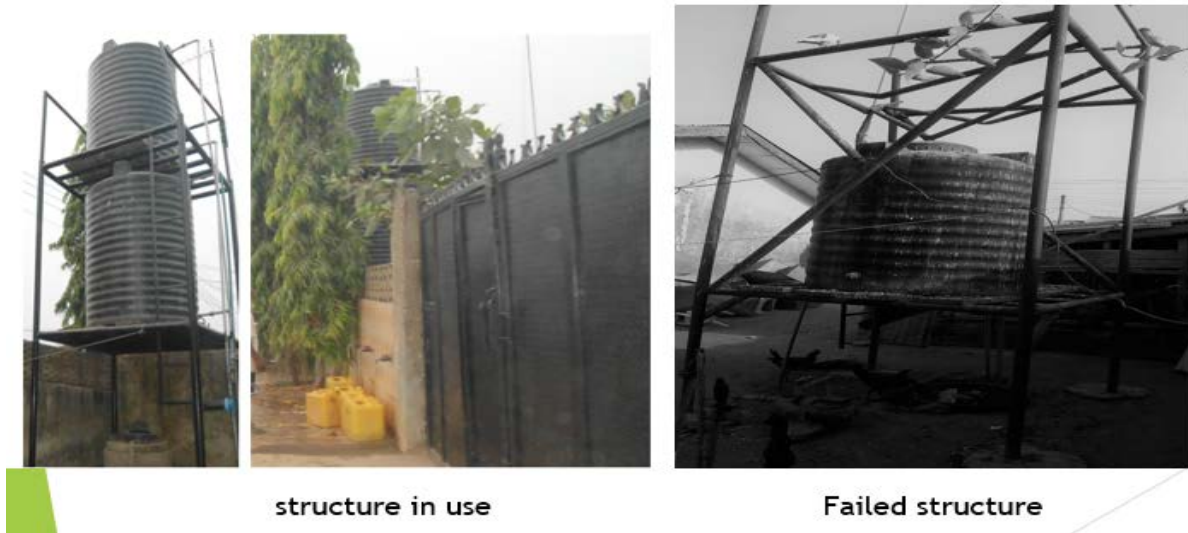
Figure 1 A household showing the overhead tank and its support in Satellite Town (Lugbe) Abuja Nigeria
