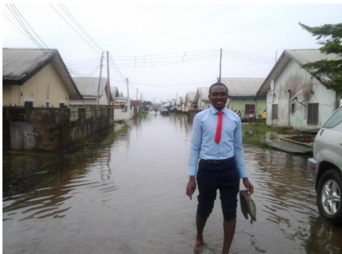
Plate 3.1: Picture showing inundation across street - Southern view of Road 2, Ekeki Housing Estate, Phase 2, Yenagoa (Photo taken on September 10, 2014)
