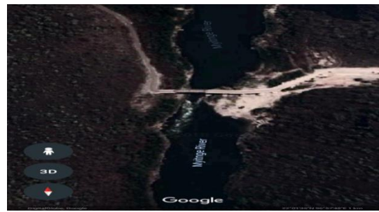
Fig. 2 Dokhtawaddy Bridge View (Source-Google)
