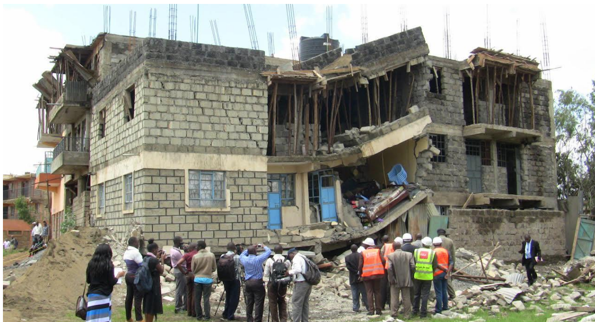
Plate 1: the debris of the building that collapsed in Kimbo area Juja Sub-County on 25th November 2016
