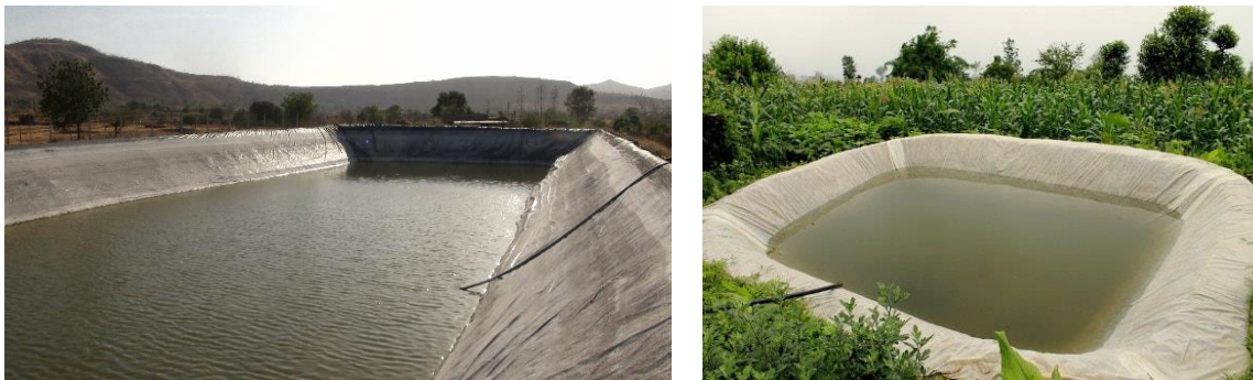
Figure 4. Concrete ponds for rainwater harvesting
