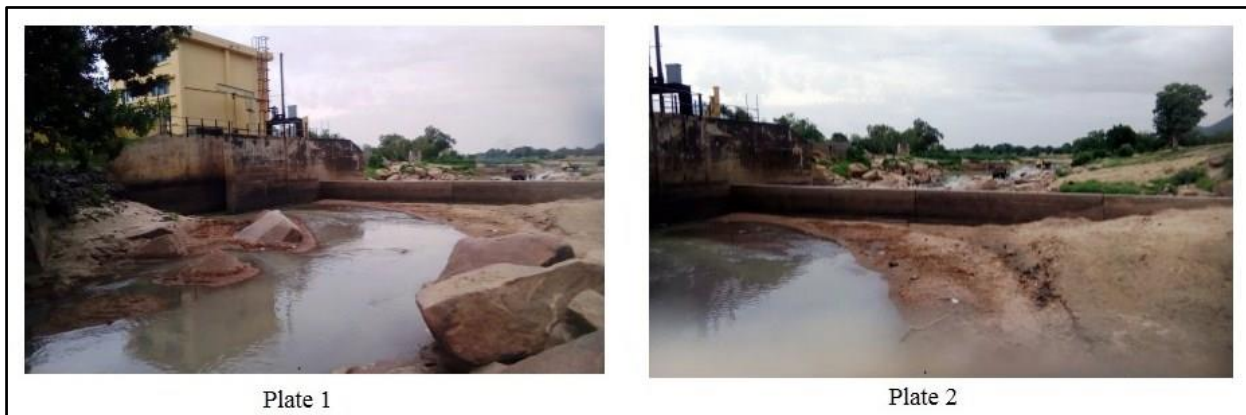
Plates 1 and 2: The barrage at Gada water treatment plant
