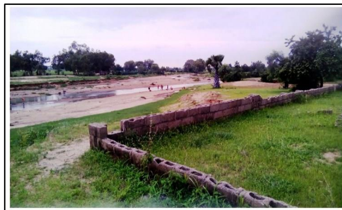
Plate 5: Bricks wall construction within the CMZ
