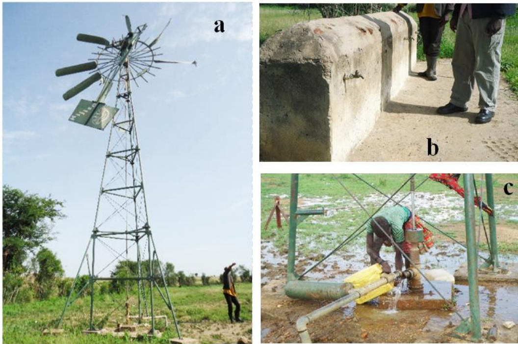
Figure 2: A non-functional windmill for water pumping (a) and tap stand (b) in Rengen Sub County. Leaking pipes at a water pumping windmill site in Lokitalebeu Sub County. All in Kotido District. Source: MoFPED - BMAI/
