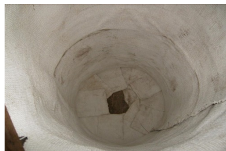
Figure 8. Covering by Asbestos Cloth
