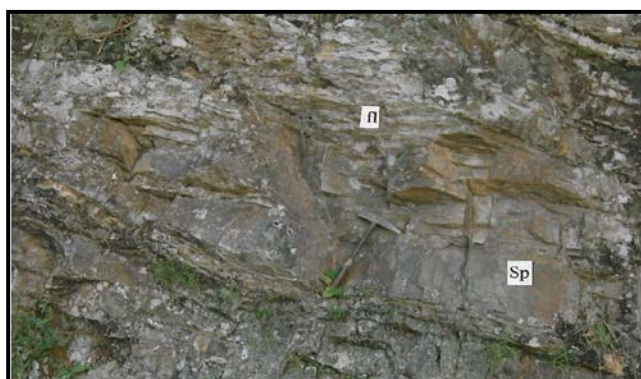
Photo 1: Well Defined Channel (0.5m across)
