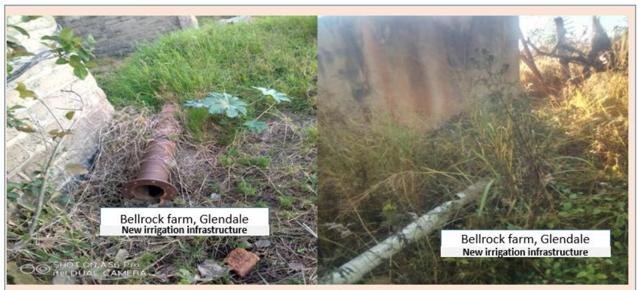
Figure 4: Vandalized irrigation infrastructure
