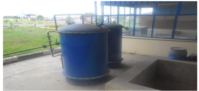
Figure 3: non-operational treatment facility
