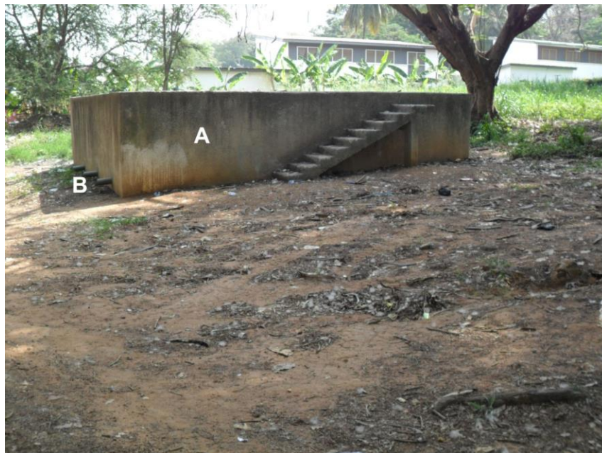
Figure 2.1: The waste site deposit: A. Four-walled concrete waste collector. B: Waste water sprout
