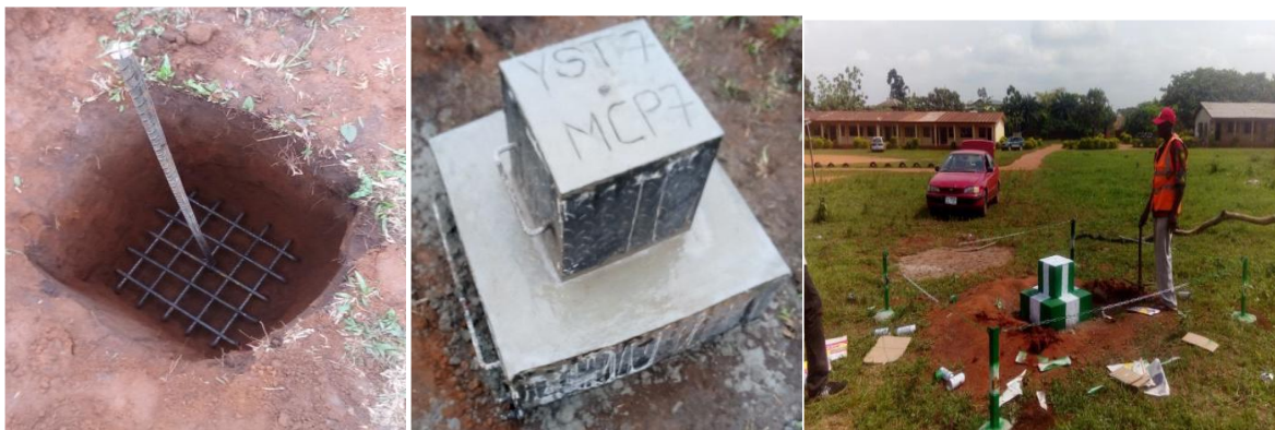
Plate 1a, b & c the constructed monitoring pillars.
