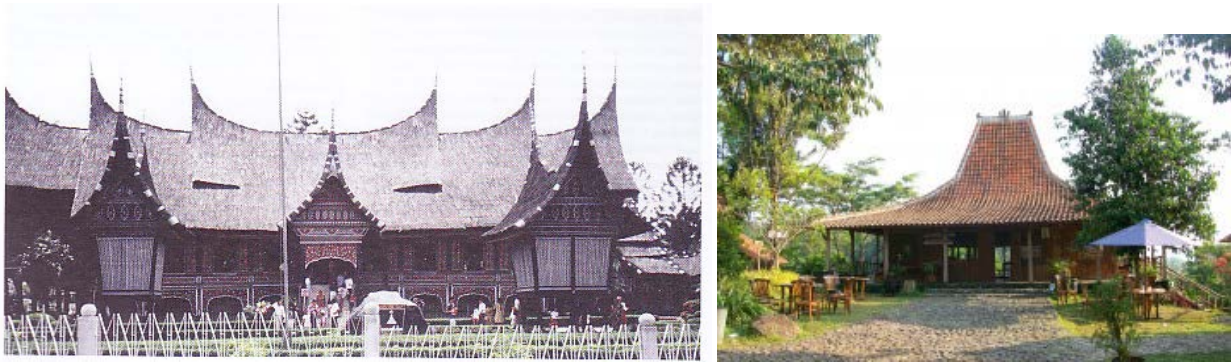
Figure 1: Rumah Gadang, Minangkabau and Joglo, Java; the examples of Indonesian traditional houses which have concerned the tropical climate. (Source: Nas, 2009, http://rumahadatkhadaerahjawa.blogspot.com/ )
