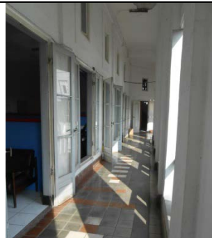
Figure 7: The corridor of Jiwasraya Insurance, as the area to penetrate solar heat and to protect from rain. The row of doors and windows are seen to support the cross ventilation inside the room. Source: private documentation.
