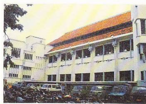
Figure 5: Mayor Office, Surabaya. Designed by an architect C. Citroen before 1927. Source: Sumalyo, 2009.
