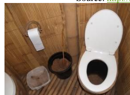
Figure 16 Composting toilet and sawdust.
