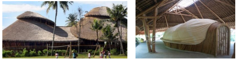
Figure 13 bubble classrooms designed to be soundproof, and the ceiling of the classroom is made of straw. Source: https://www.flickrriver.com/photos/gregersreimann/sets/72157623535475431
