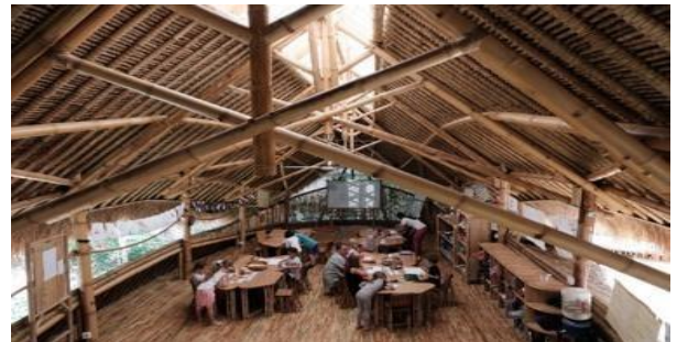
Figure 1 Perspective View of Interior of Green School Bali, Showing the Use of Bamboo
