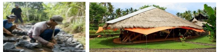
Figure 11 Showing the pavement and pathways. Source: https://www.ted.com/talks/john_hardy_my_green_school_dream
