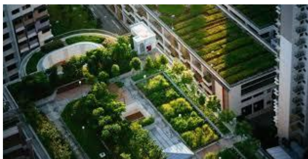
Figure 4: showing a green roof. Adapted [36]
