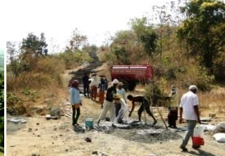
Construction in forest area
