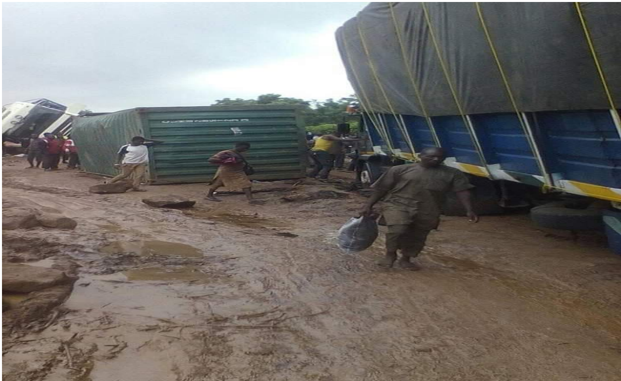
Fig 1: Failed portion of road resulting to delay in travel time
