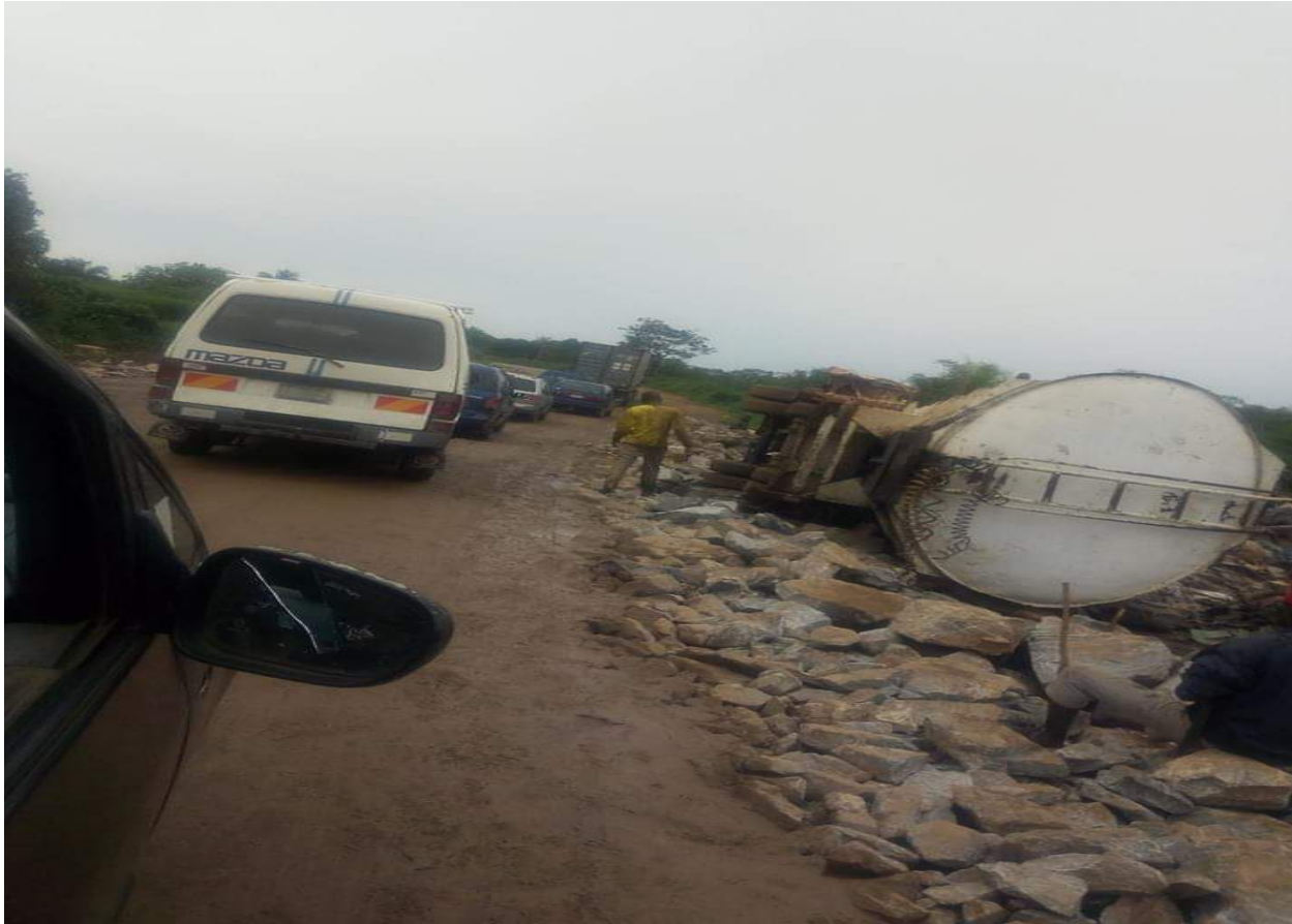
Fig 3: Overturned truck as a result of failed spots on the road
