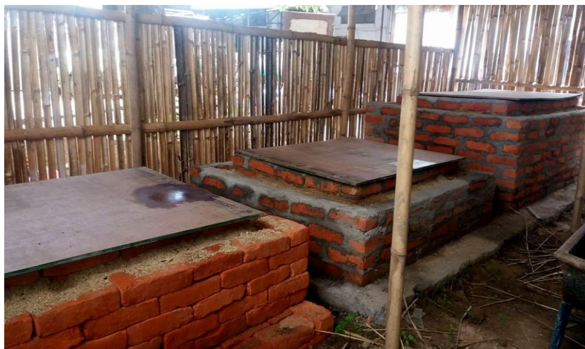
Fig. 1: Photographic view of Zero energy cool chamber (ZECC) constructed at Agricultural Engineering Division, Khumaltar.
