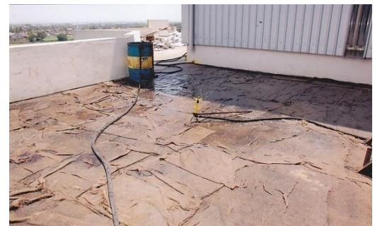
Fig 3: Water Sprinkler used for plain area.
