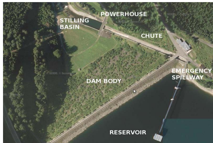
Figure 1: Overhead view of the right abutment of the Sance Dam
