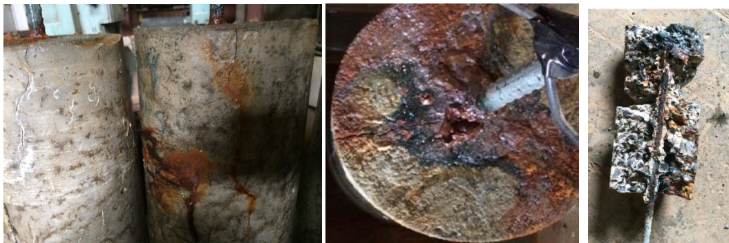
Figure 3.4 Images of corrosion samples after corrosion.
