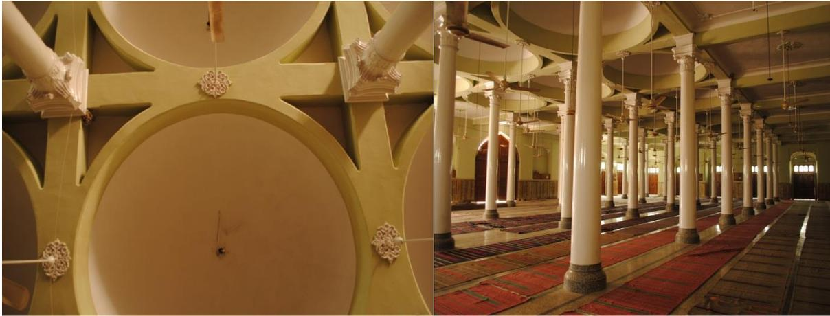
The roof of the chamber is supported by means of thirty-two columns finished in white marble. The curved space is divided into horizontal north-south strips by inverted beams. Twenty-one
