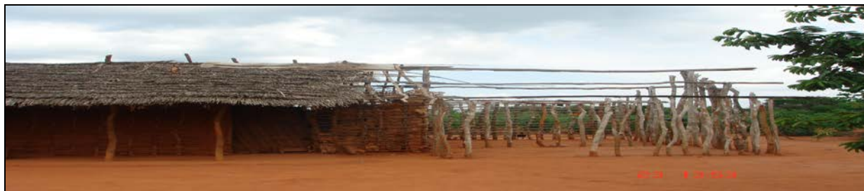
Figure 2: A thatch-roofed house built with small poles and mud reflecting reliance on Mother Nature in Vibura sub-village in Kazimzumbwi village
