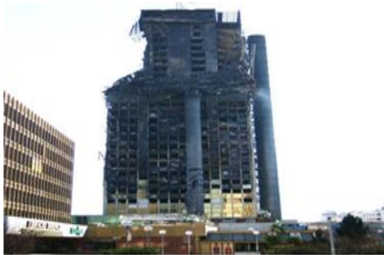
Figure 1.1: The Windsor Tower in Madrid after a 26 hour fire in 2005.
