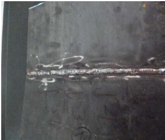
Figure 1: Image of Normal Welding of 4mm Thick Plates
