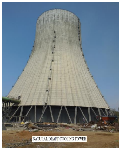
Figure 1: Natural draft cooling tower
