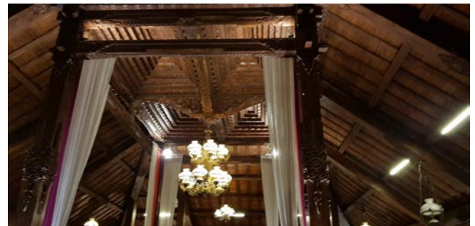
Figure 12. 2nd Floor Ceiling Detail
