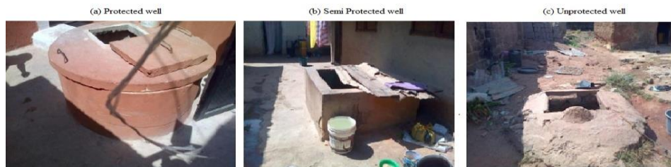
Figure 1: Hand dug wells in Hardo ward. Sources of water pollution in hand dug wells (HDW)
