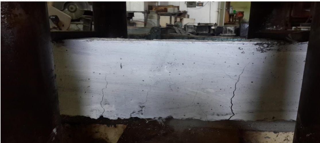
Figure 7: Appearance of cracks at failure
