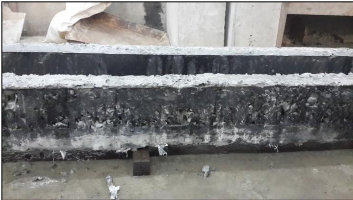
Figure 13: Honeycombs on the dry bamboo beam sample
