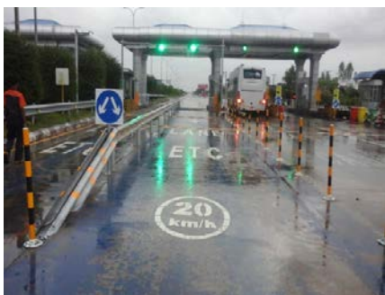
Figure 11. ETC Lane of No.3 Joint at Yangon-Mandalay High Way
