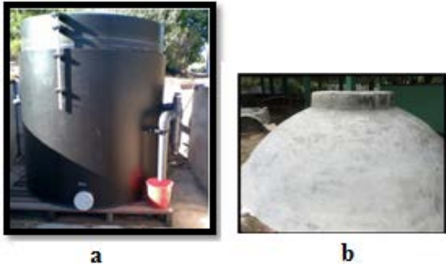
Figure 2: (a) Floating-drum biogas plant using 15000 liter water tank (b) Ferro cement biogas plant at Mahadeva Achchiramam - Killinochi
