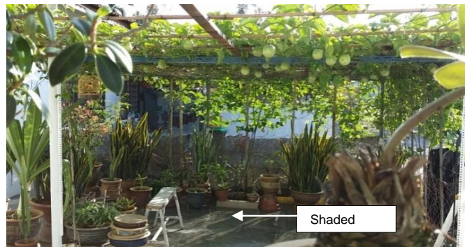
Fig. 4 Vegetated trellises grown climbing plants as a roof canopy to reduce solar energy collected by the ground surface. Source: Author
