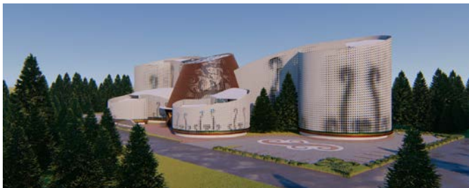
Fig. 20. The look of the building that shows the shape of the kawit carving
