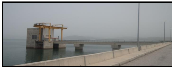
Plate III: Bottom Outlet Structure of Gurara Dam
