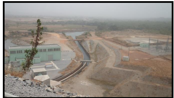
Plate V: The Power House and Switch Yard of Gurara Dam
