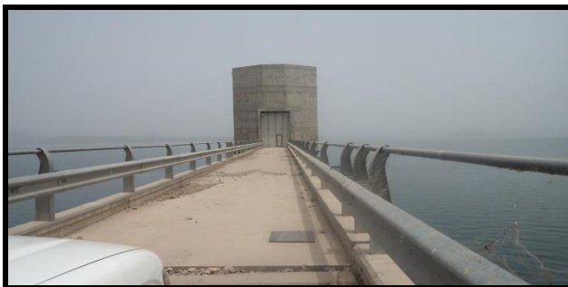
Plate VI: Pipeline Intake and Tunnel of Gurara Dam
