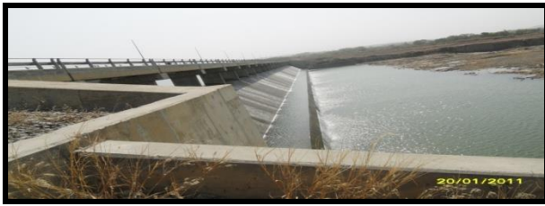
Plate II: Spillway/Stilling Basin of Gurara Dam
